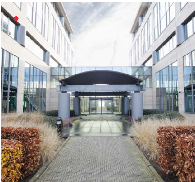
Park Lane office building – Brussels periphery (BE)
