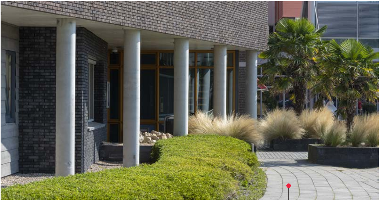
Medical office building Sionsberg – Dokkum (NL)
