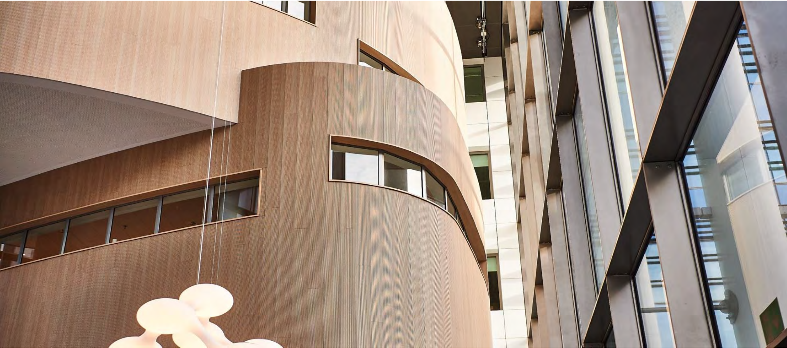
Belliard 40 office building – Brussels CBD
