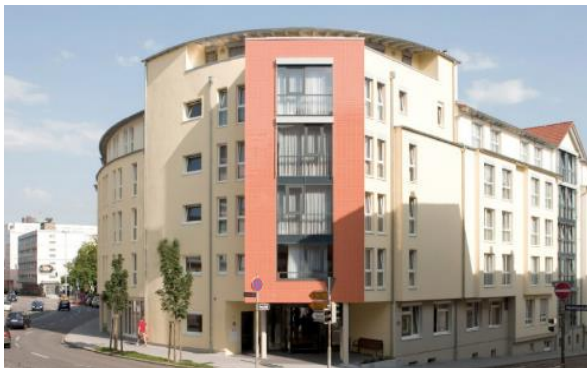
Nursing and care home Haus Osterfeld – Pforzheim
