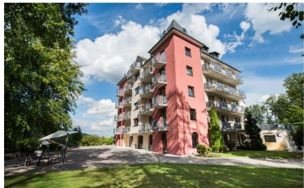
Nursing and care home Parkhöhe – Lindenfels
